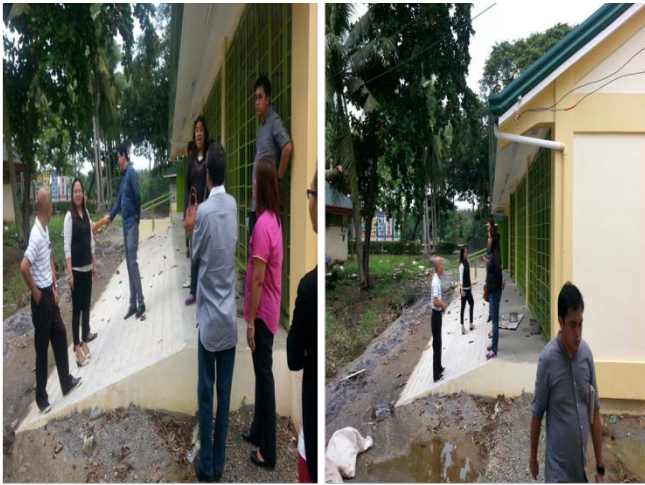
CY 2015 CONSTRUCTION OF LABORATORY WORKSHOP- MALOLOS MARINE FISHERY SCHOOL & LABORATORY
