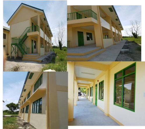
CY 2014 CONSTRUCTION OF 2 STY. 4CL- MALOLOS MARINE FISHERY SCHOOL & LABORATORY
