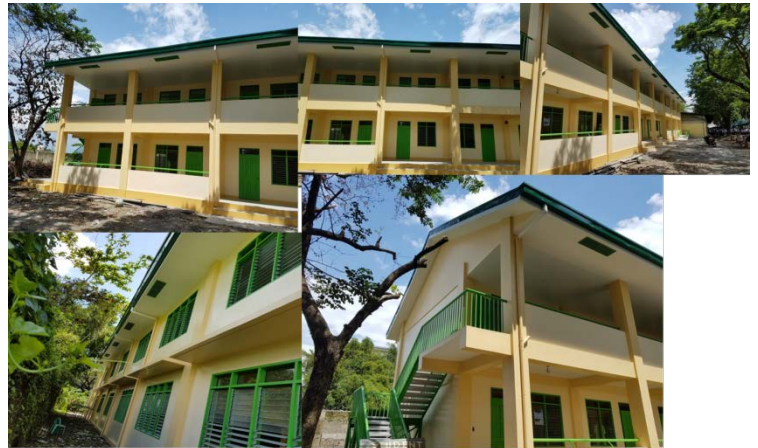
CY 2015 CONSTRUCTION OF 2 STY. 6CL FOR SHS- MARCELO H. DEL PILAR NATIONAL HIGH SCHOOL
